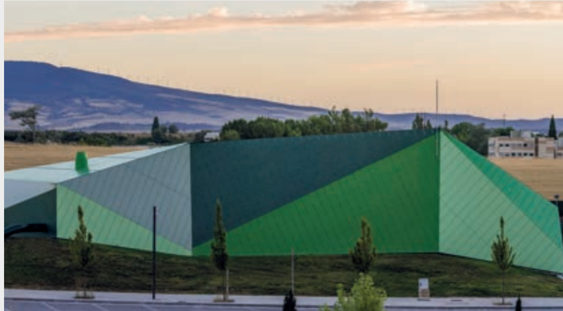
Waste collection station/terminal at Lezkairu, Pamplona, Spain
