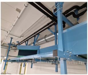
for waste disposal, and touch screens are conveniently located beside them for monitoring and control. In the basement, the technical area features solidly constructed conveyors that guide general waste sacks into separate containers for recycling. This advanced waste management system improves the hospital's overall cleanliness and sanitation while promoting sustainability efforts through the recycling of materials.
